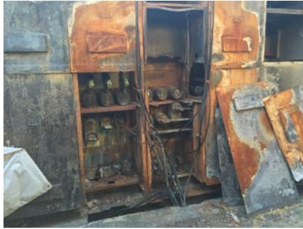
**Excessive Temperature.** Circuit breaker, bus bar, and cable connections tend to loosen and/or corrode over time, resulting in thermal failure of the connection and nearby cable insulation.
