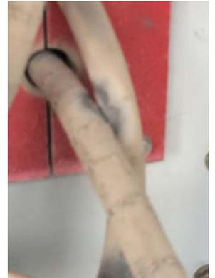
**Visually confirmed PD in a 13.8KV generator.**
